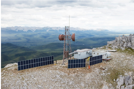
Solar-diesel hybrid power generation with Northwestel. Photo credit: Fritz Mueller
